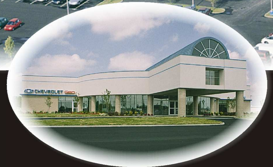
Central Chevrolet; B. B. Vance & Sons, Inc., builder; Little & Maddox Architects.
