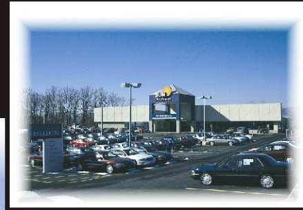
Sun Auto Group; B. K. Structural Systems, builder; John Gianacopoulos, architect.
