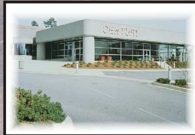
Century Acura; R. T. Murrell Const. Co., Inc., builder; Design Collaborative, architect.
